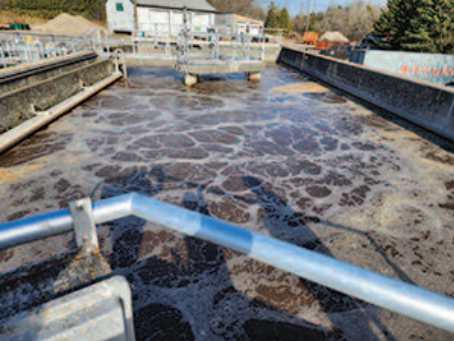
An aeration pond at the Uxbridge Brook Water Pollution Control Plant, the site for secondary wastewater treatment.
